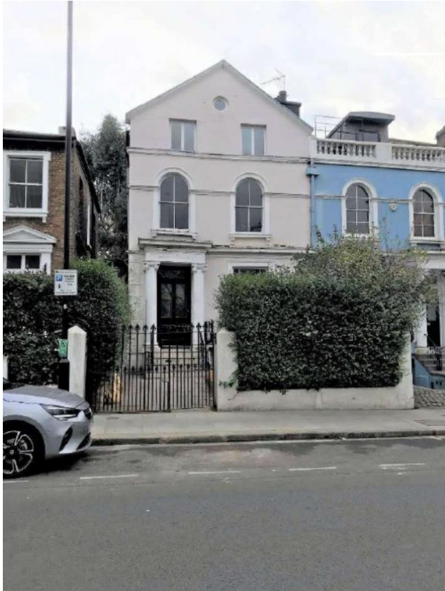
Photo of pre-existing front elevation
